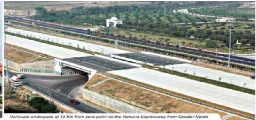
Vehicular underpass at 12 Km from zero point on the Yamuna Expressway from Greater Noida
